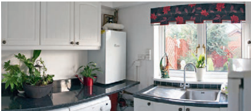
Bottom: The boiler takes up little space in the home.
