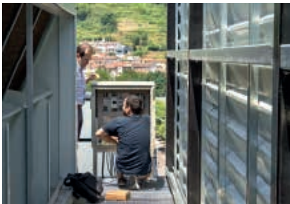
A team from Intersam, Fritecno and ebm-papst inspecting the abattoir heat exchangers in operation
