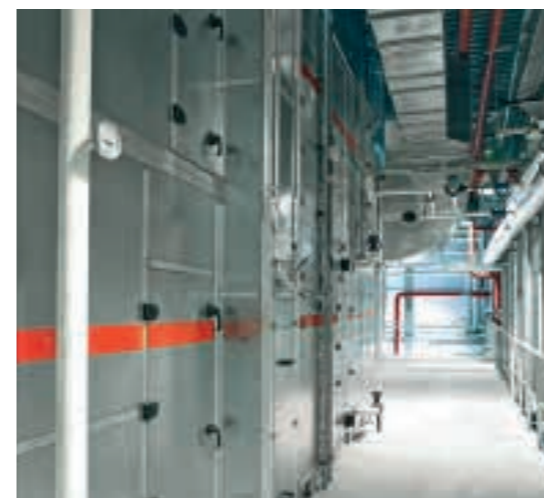
Left: The Thermobloc central climate control units are installed in the Moskvarium's cellar.
