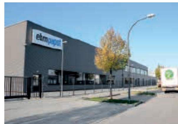
Since September 2015, Plant 2 in Landshut provides the capacity required for producing efficient gas blowers and valves.
