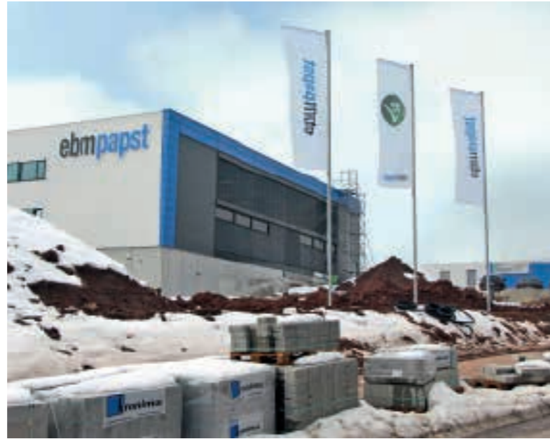
The completed first phase of construction in St. Georgen-Hagenmoos
