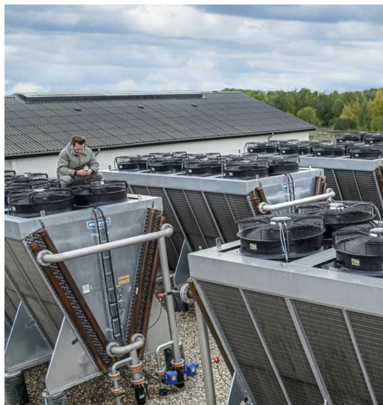
Whether spring, summer or autumn — the 80 AxiBlade EC fans work in every season. They can even cope with ice.
