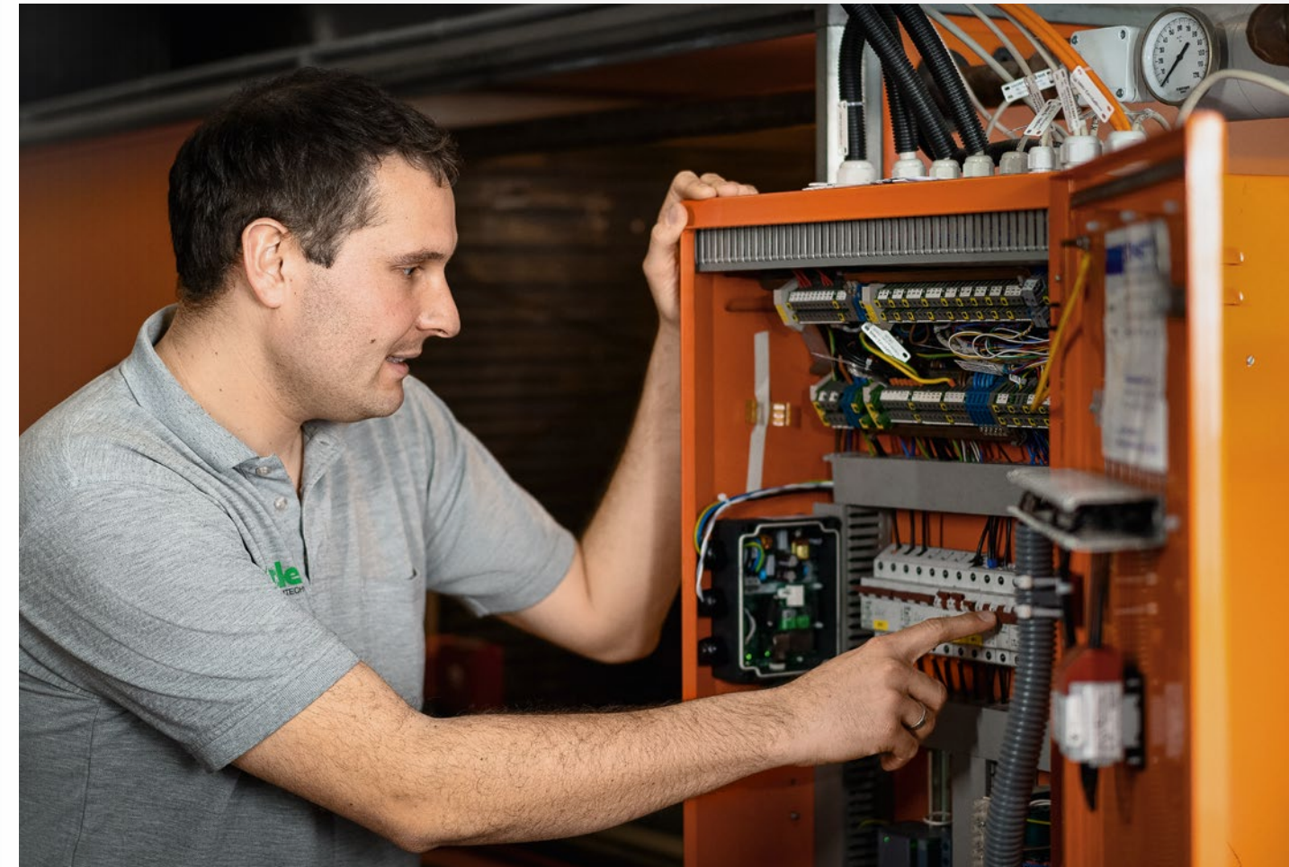
The system’s control cabinet was still in good condition. It was modernized, including a new control and an ebm-papst neo gateway. Instead of the old belt-driven fans, eight new RadiFit centrifugal fans now provide fresh air.
