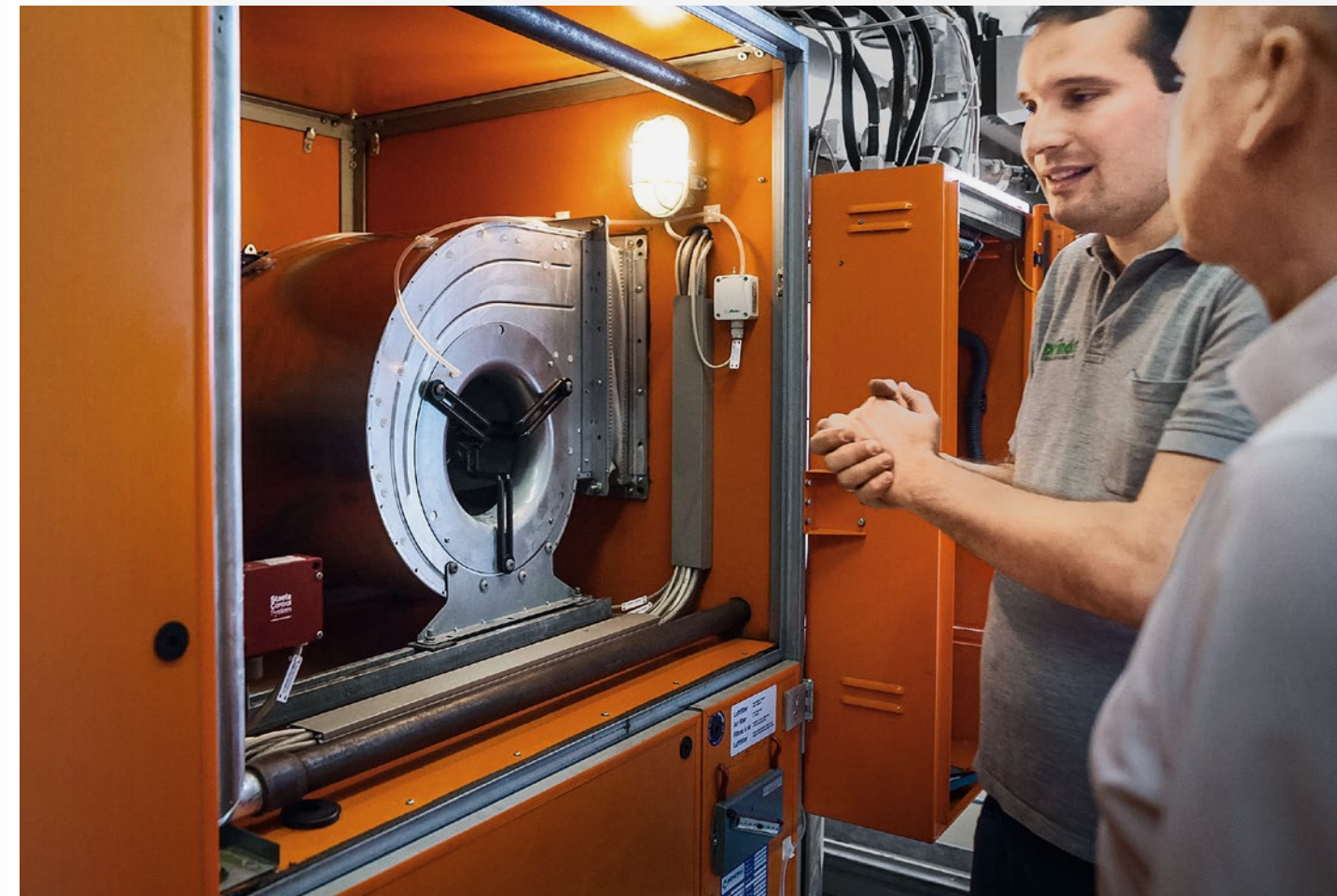
The system’s control cabinet was still in good condition. It was modernized, including a new control and an ebm-papst neo gateway. Instead of the old belt-driven fans, eight new RadiFit centrifugal fans now provide fresh air.
