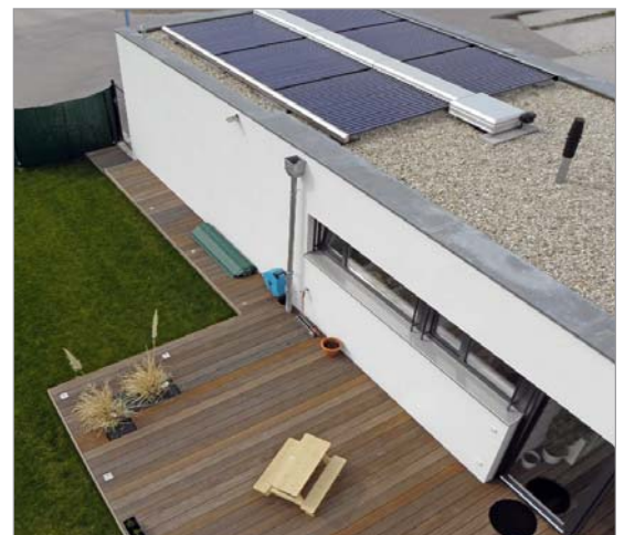
Figure 3: Sun-Storm collector on the flat roof of a single-family home (photo: Kollektorfabrik)
