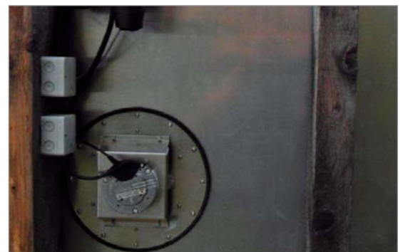
Figure 4: The liquid air box (viewed from the rear) with heat exchanger and fan impresses with its compact dimensions. (photo: Kollektorfabrik)
