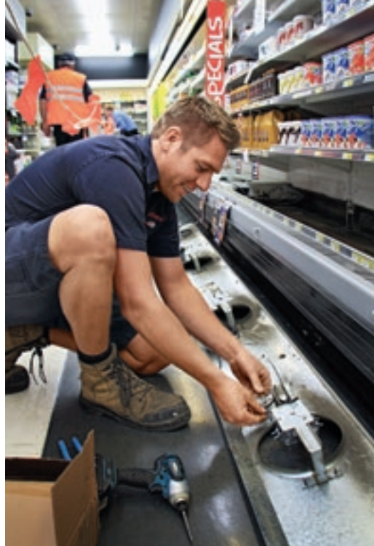
Replacement in only 15 minutes: Neal Murtagh replaces outdated AC technology with energy-saving iQ-motors with GreenTech EC technology
